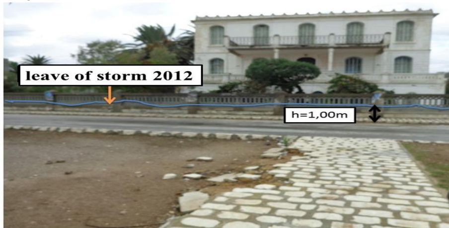
Figure 5. Schematic of the 2012 storm leash in Hammam Lif and the water depth marked on a house wall
