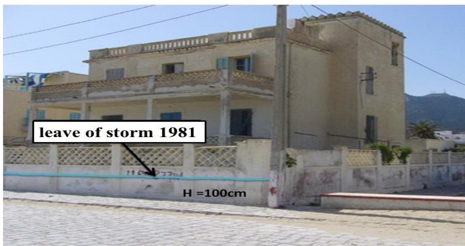
Figure 3. Diagram of the 1981 Storm Leash at Hammam Lif and the water depth marked on a wall of a house
