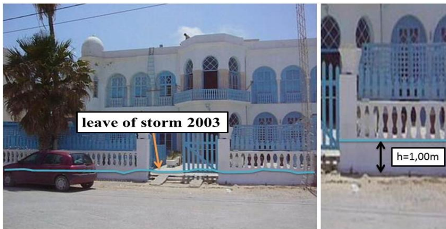
Figure 4. Schematic of the 2003 storm leash at Hammam Lif and the water depth marked on a house wall
