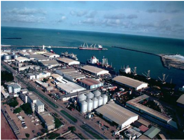
Figure 1: Partial view of the facilities of the Port of Cotonou
